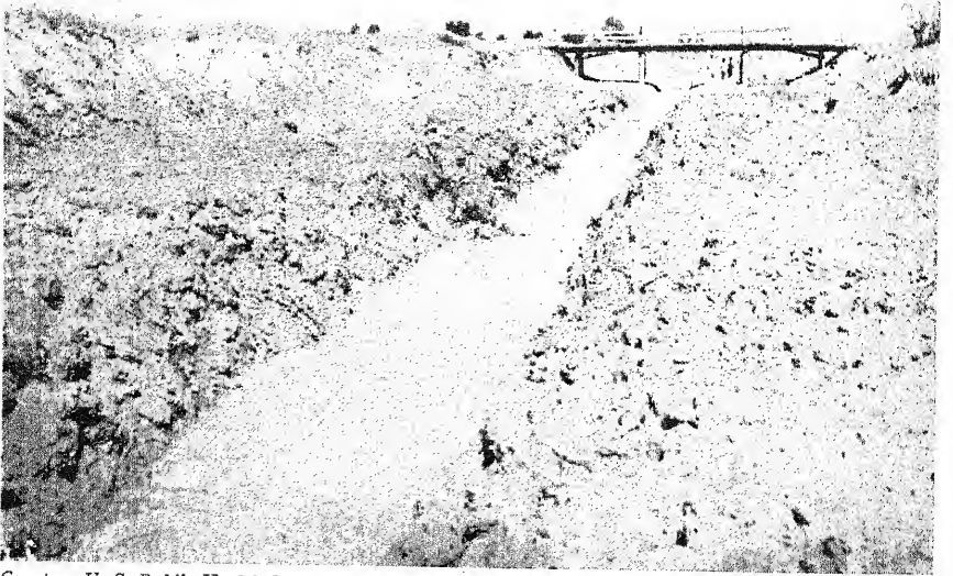
Figure 27. Drain deepened by blasting with dynamite
